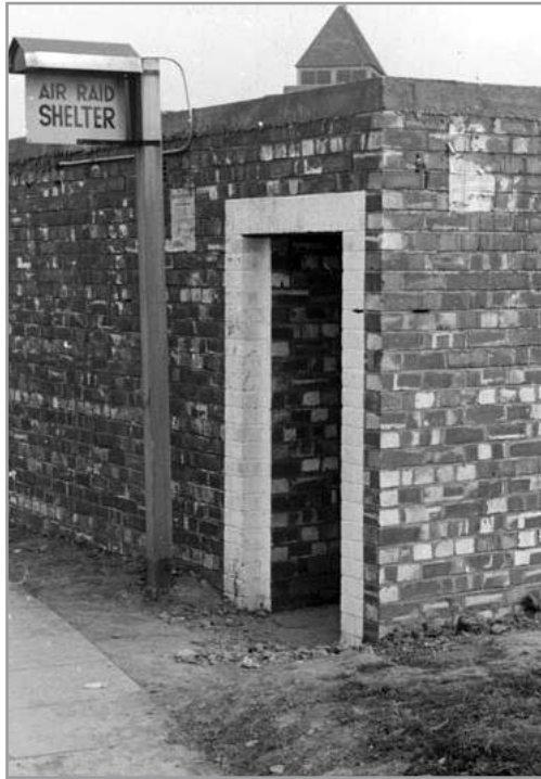
a shelter of the similar brick and concrete construction as those used in the area
